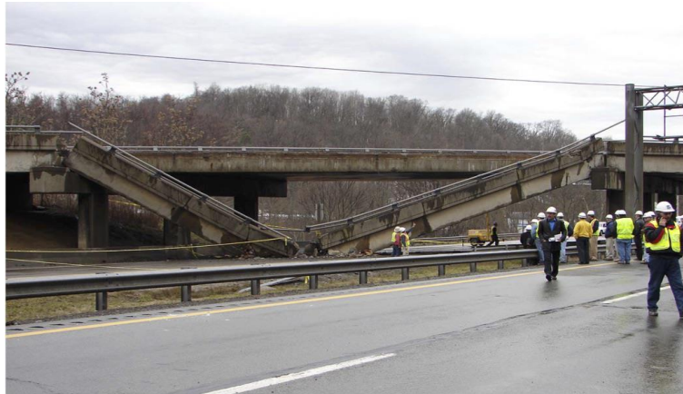
Abb. 1: Einsturz Lake View Drive Bridge am 27.12.2005
